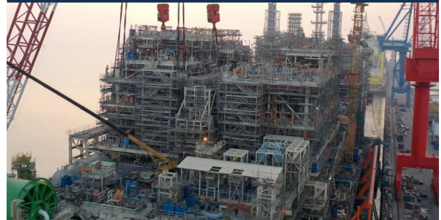
FPSO – Topsides Installation
