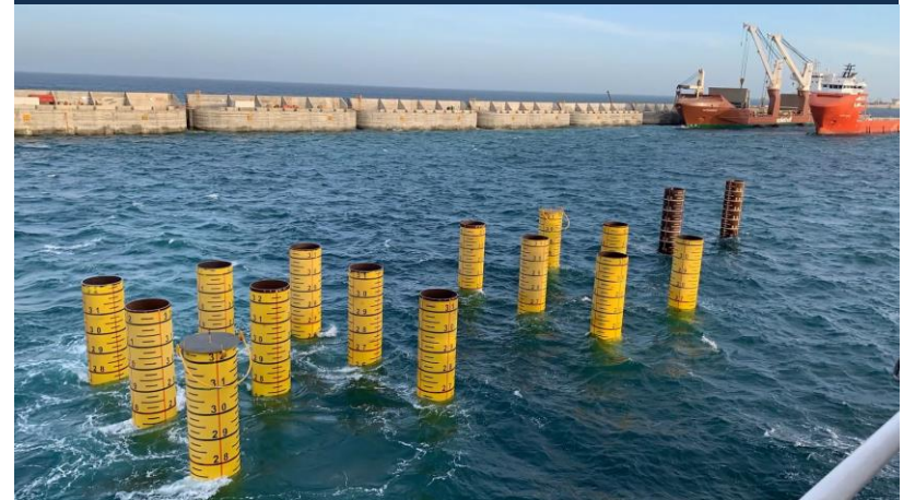
Hub Terminal – Jetty Piling
